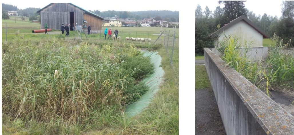
Figure 1: Examples of RB units operated as part of a small WWTP in the Waldviertel region of Austria (Autumn 2017)
